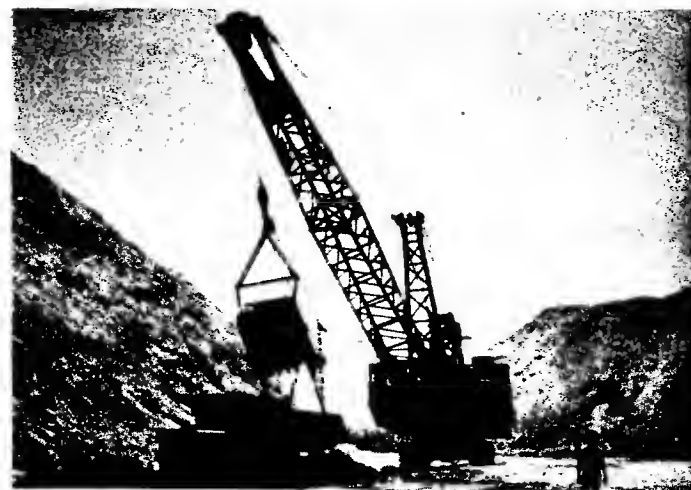
FIG. 1.4 Open cast mining in Morocco.
