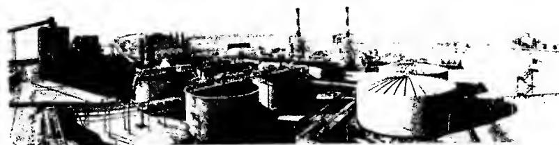
FIG. 1.2 Overall view of SAEPA complex producing phosphoric acid in Gabes, Tunisia. (Courtesy of Heurtey Industries, Paris, 1979.)
