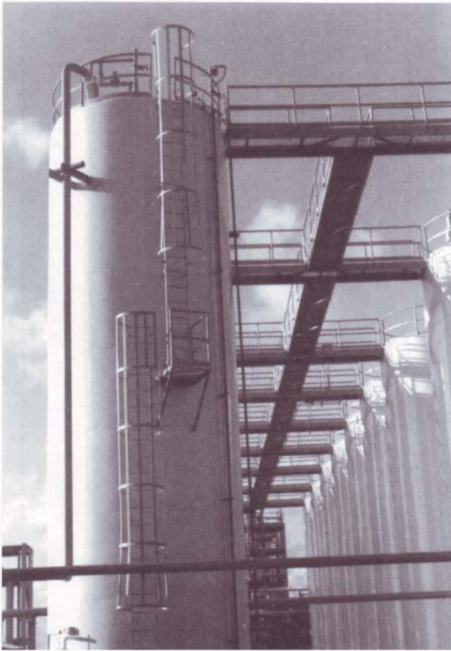
FIGURE 6.9 Ladder, cage, and platforms. Courtesy of Nisseki Chemical Texas, Inc., Bayport, Texas.
