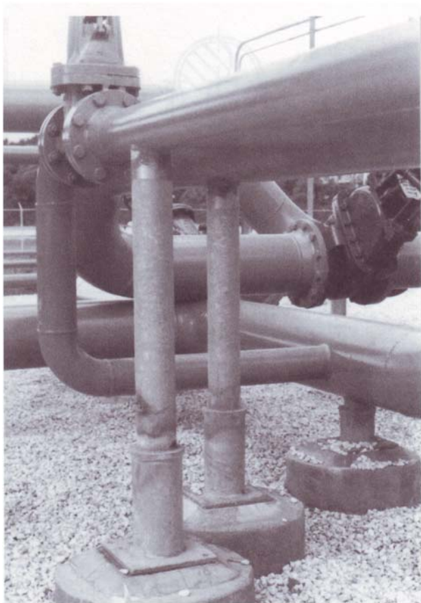
FIGURE 11.17 Field support. Courtesy Nisseki Chemical Texas, Inc., Bayport, Texas.
