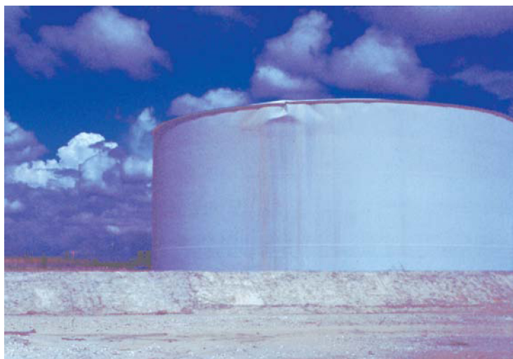
Figure 2.12 Large tank (100-ft. diameter) damaged by overfilling.
