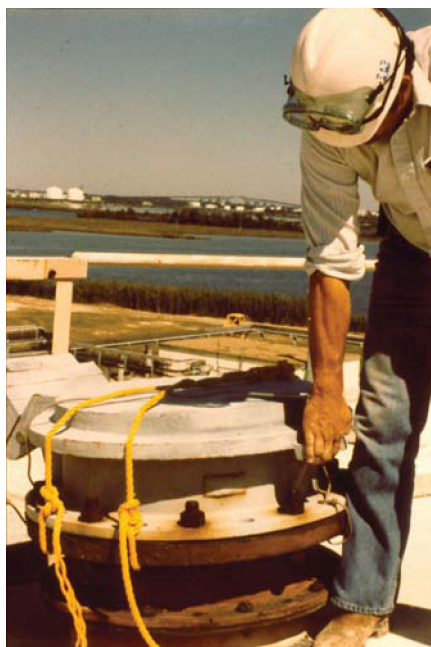
Figure 8.12 Hinged vent lid improperly tied to cope with anticipated high winds and to prevent intrusion of rain during the threat of a hurricane.
