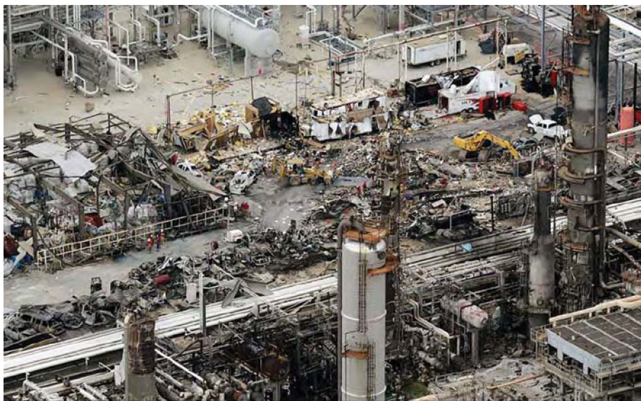
Figure 4.7 Aerial view of the destroyed trailers near the ISOM area after the explosion and fire. Photo Courtesy of CSB Report No 2005-04-1-TX and was on the cover of the report.
