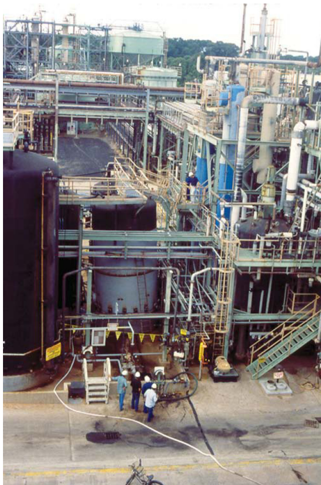
Figure 3.1 An API 620 tank is damaged during a hydro-test that went awry.
