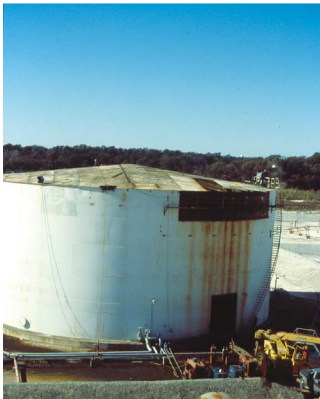
Figure 8.14 Repairs in progress on a large API – 650 tank.
