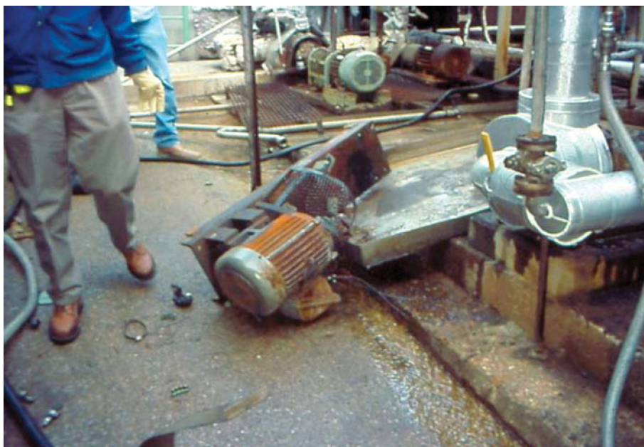
Figure 9.15 Pump base plate and motor propelled from operating position into the walkway. Courtesy of Eastman Chemical Company.
