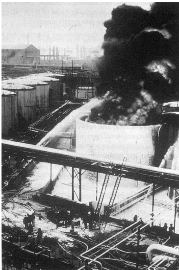
Figure 10.5 A tank fire confined by tank walls in a floating roof crude oil tank. Courtesy of the Institution of Chemical Engineers – from Hazard Workshop No. 6, “Preventing Emergencies in the Process Industries, Vol. 1.”
