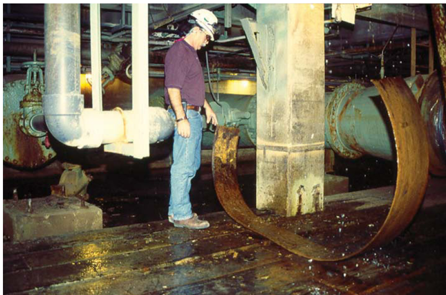
Figure 9.12 The force of the explosion reshaped and straightened a portion of the 42 in. diameter Dresser coupling.
