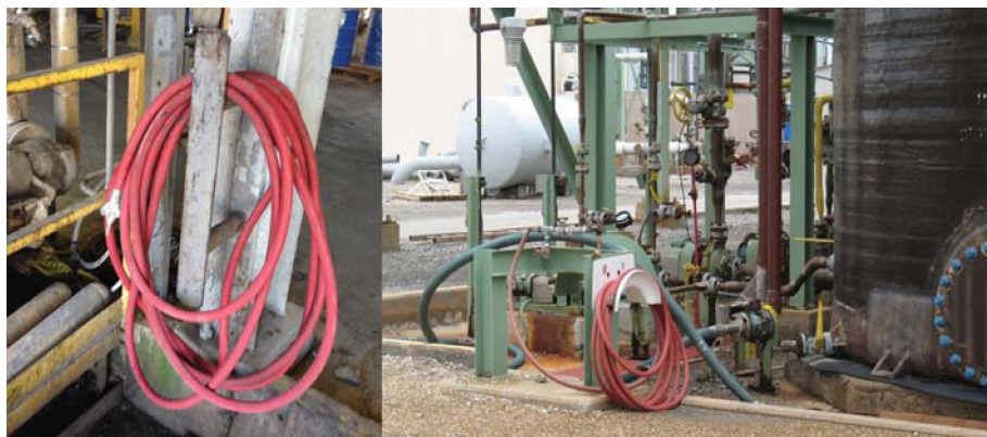
Figure 9.5 Hoses are indispensable and ever present in most chemical plants. A British study over an 11 year period found hoses were involved in about 10% of all loss of containment incidents.
