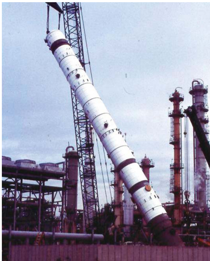
Figure 12.1 Mechanical integrity starts long before the equipment is being installed. Mechanical integrity starts with the design to appropriate codes, the fabrication to standards and the testing to codes. Mechanical integrity continues with routine inspections and tests per codes as well as maintenance. MI does not end until the equipment is taken out of service.
