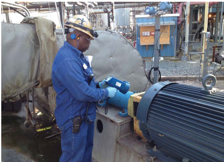
Figure 12.4 A mechanic is inspecting a blower coupling condition and alignment using a timing light at a specialty chemical facility.
