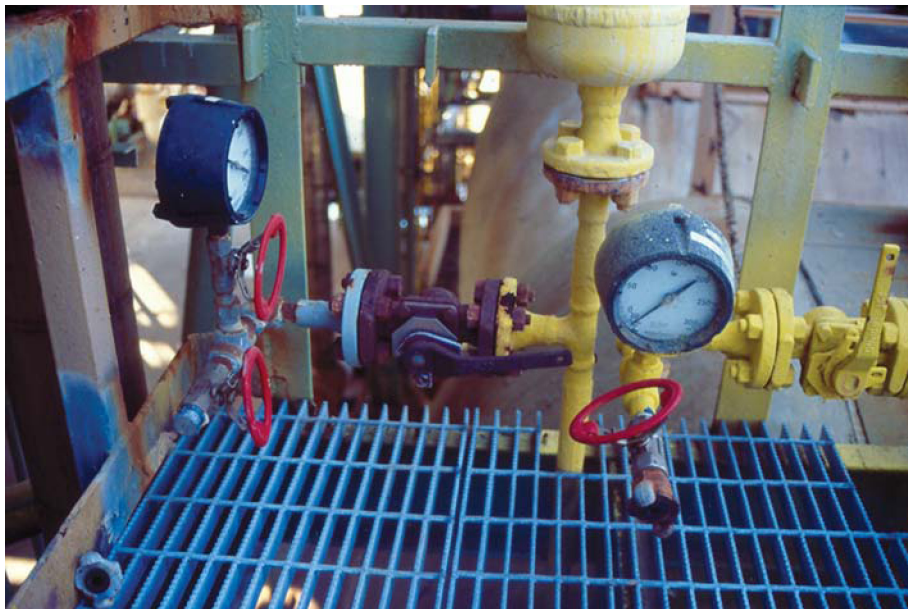
Figure 9.8 Close-up of piping arrangement reveal that the hose connection for the middle expansion bottle is in front of the south bottle. Furthermore, the lack of paint on the small piping to south expansion bottle sort of camouflages the piping under dim lighting of the night.
