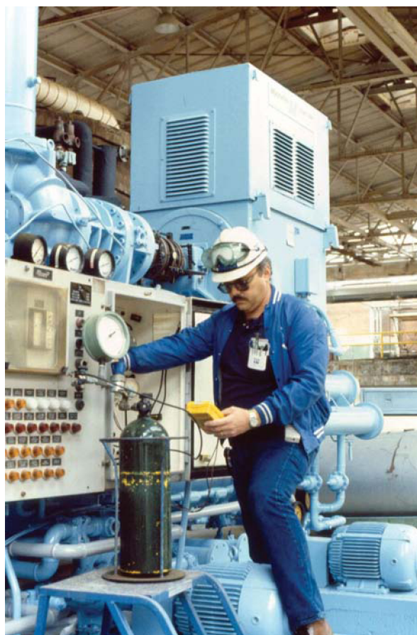
Figure 12.28 Proof testing a high-pressure switch on a large refrigeration unit.
