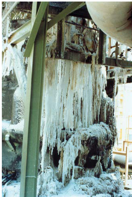
Figure 8.8 Chemical icicles are formed from a small caustic soda leak that dripped from an evaporator flange.
