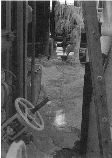
Figure 8.7 Molten caustic leaks from above due to an improper gasket.
