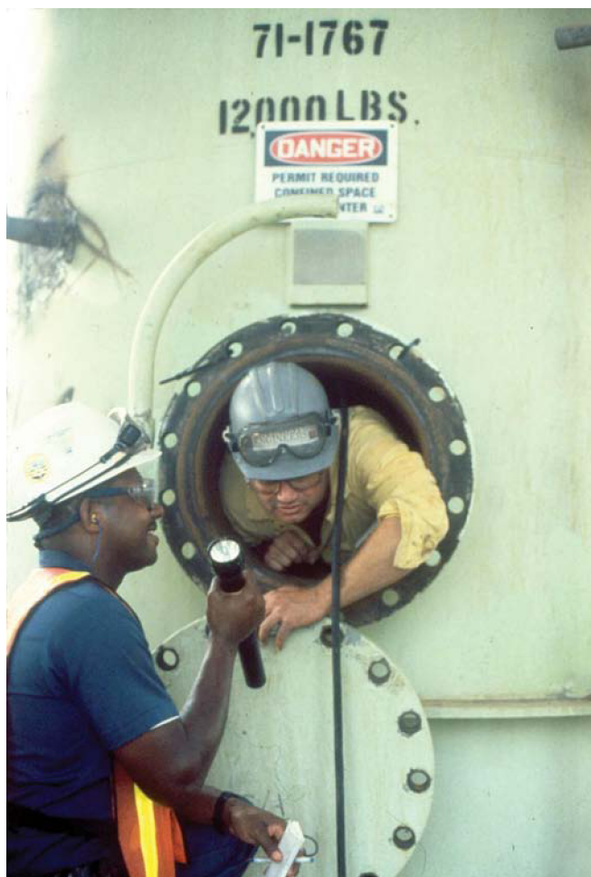
Figure 12.12 A certified pressure vessel inspector enters the confined space after the vessel is cleared, blinded, and tested. However another employee (a manway watch) must be in place outside the vessel with emergency communications equipment.
