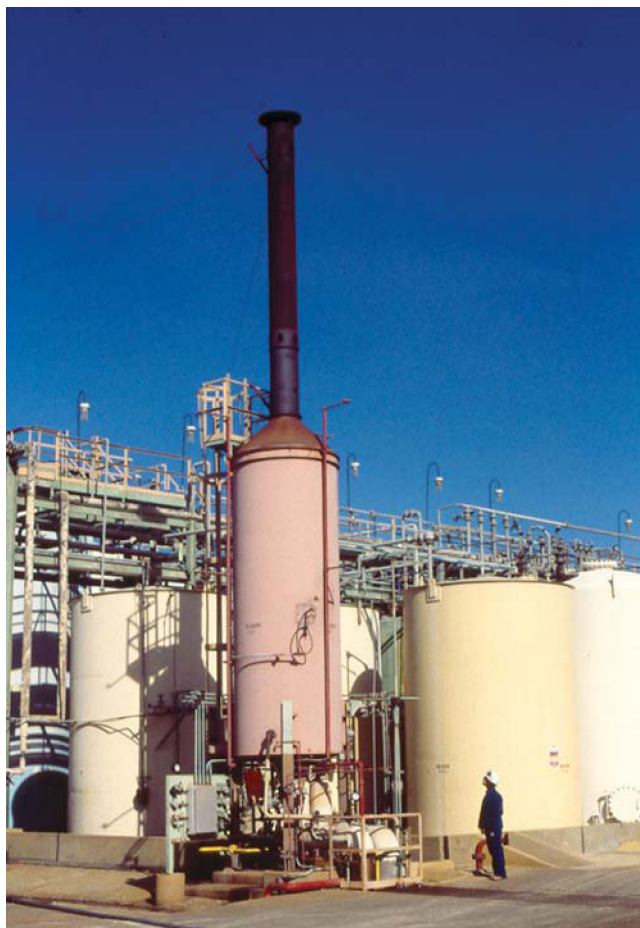
Figure 8.5 The re-built gas-fired heater was relocated away from the process area and the hard to replace process equipment and instruments.
