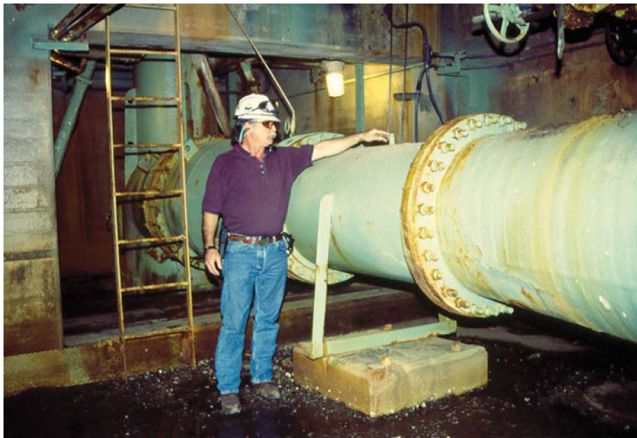
Figure 9.9 A view of an identical river water pump discharge piping that was adjacent to the pump that experienced an explosion.
