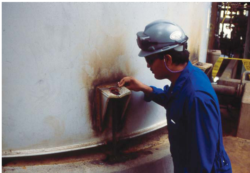
Figure 3.4 Tank bottom is bulged and anchor bolt nuts are pulled through the anchor chairs.
