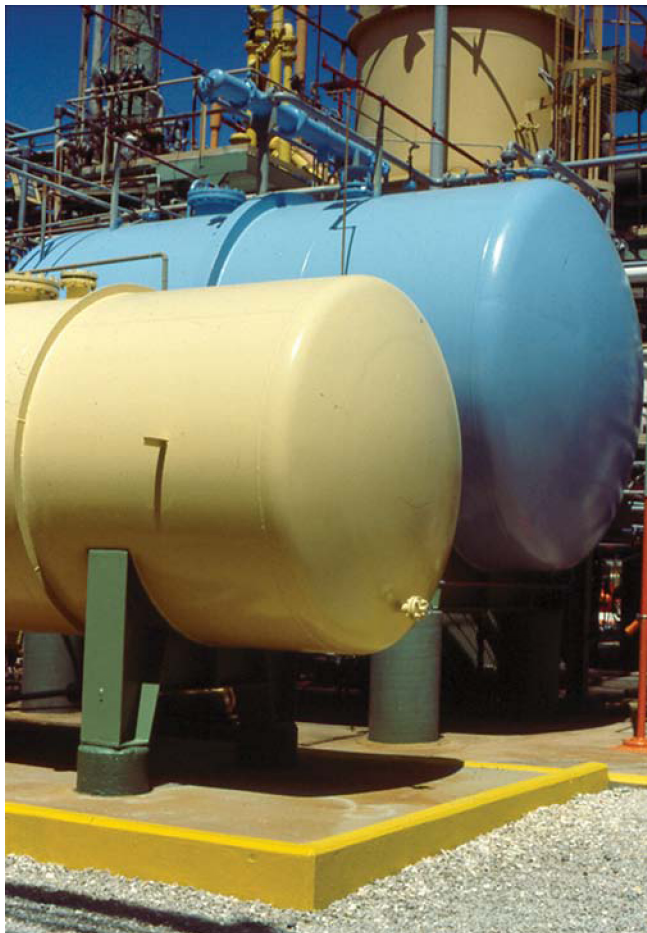
Figure 12.9 Well-maintained pressure vessels (over 40 years old) still safely handling hazardous solvents and with proper management it will last another 40 years.
