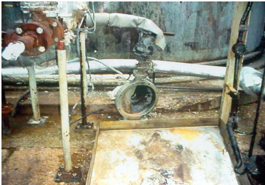
Figure 9.14 Pump bowl is stripped of the pump and base plate. Courtesy of Eastman Chemical Company.
