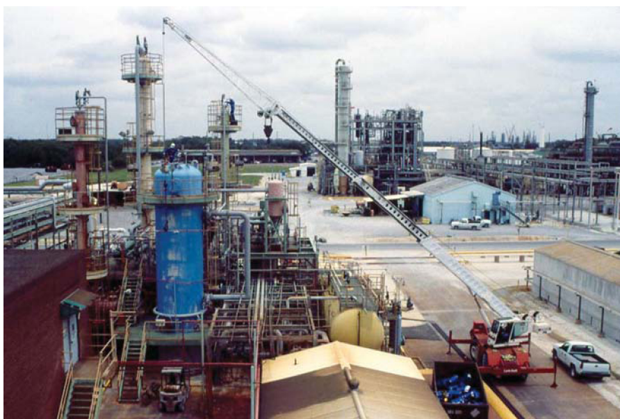
Figure 12.24 A crane is reaching out and lifting a recently tested and reconditioned safety relief valve to reinstall on a reactor.
