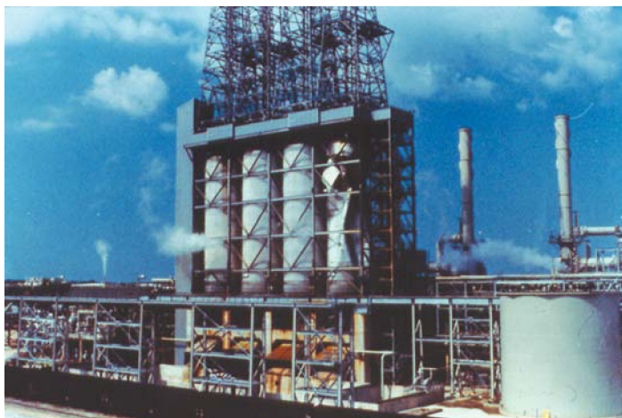
Figure 3.11 Coker Drum destroyed - crushed in like an aluminum beer can. Courtesy of S.O. Kapenieks.
