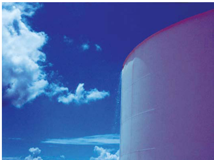
Figure 2.11 Liquid product spilling from the roof seam of a damaged tank.
