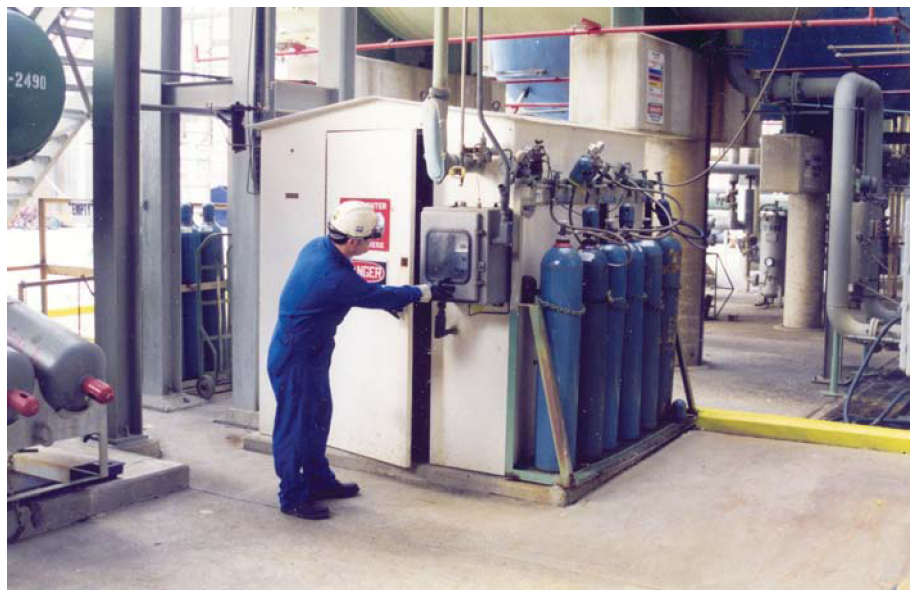
Figure 2.23 Typical pressurized and purged analyzer buildings found in chemical plants handling flammables.
