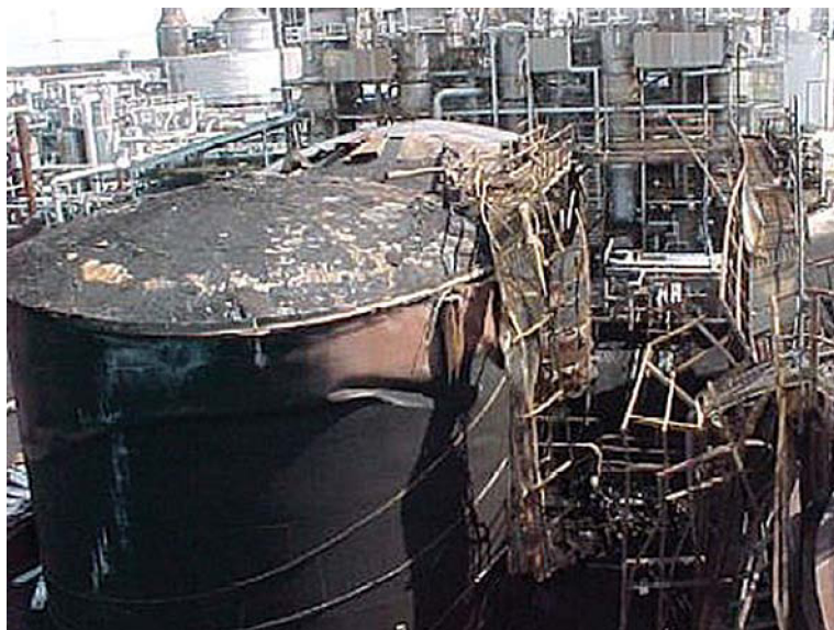
Figure 7.5 Charred sulfuric acid Tank No. 394 in foreground and the remains of the catwalk on the right.
