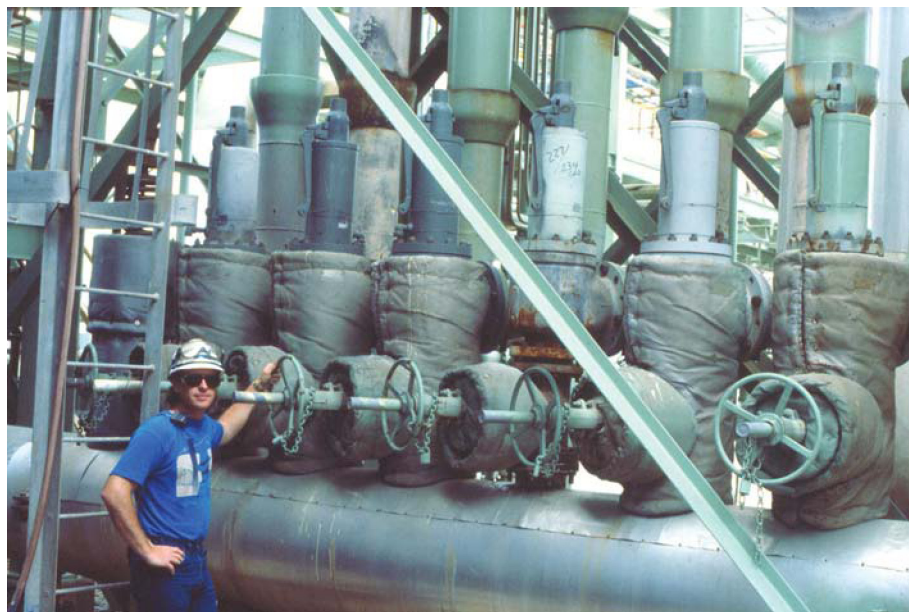
Figure 12.26 A powerhouse operator relies on a bank of large safety relief valves to protect equipment and personnel at this location.
