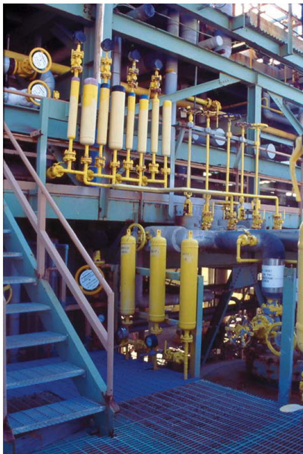
Figure 9.7 Chlorine expansion bottles per the chlorine institute protecting chlorine transfer piping from overpressure.
