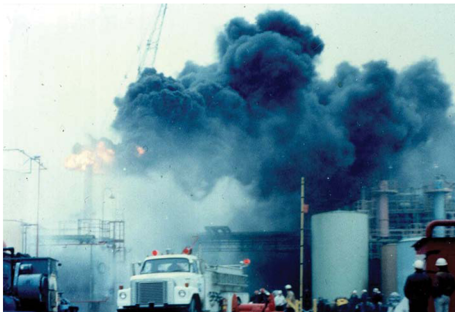
Figure 10.2 Fired heater tubes frozen – improperly thawed – tubes ruptured – heat transfer fluid burns – emergency squad responds.
