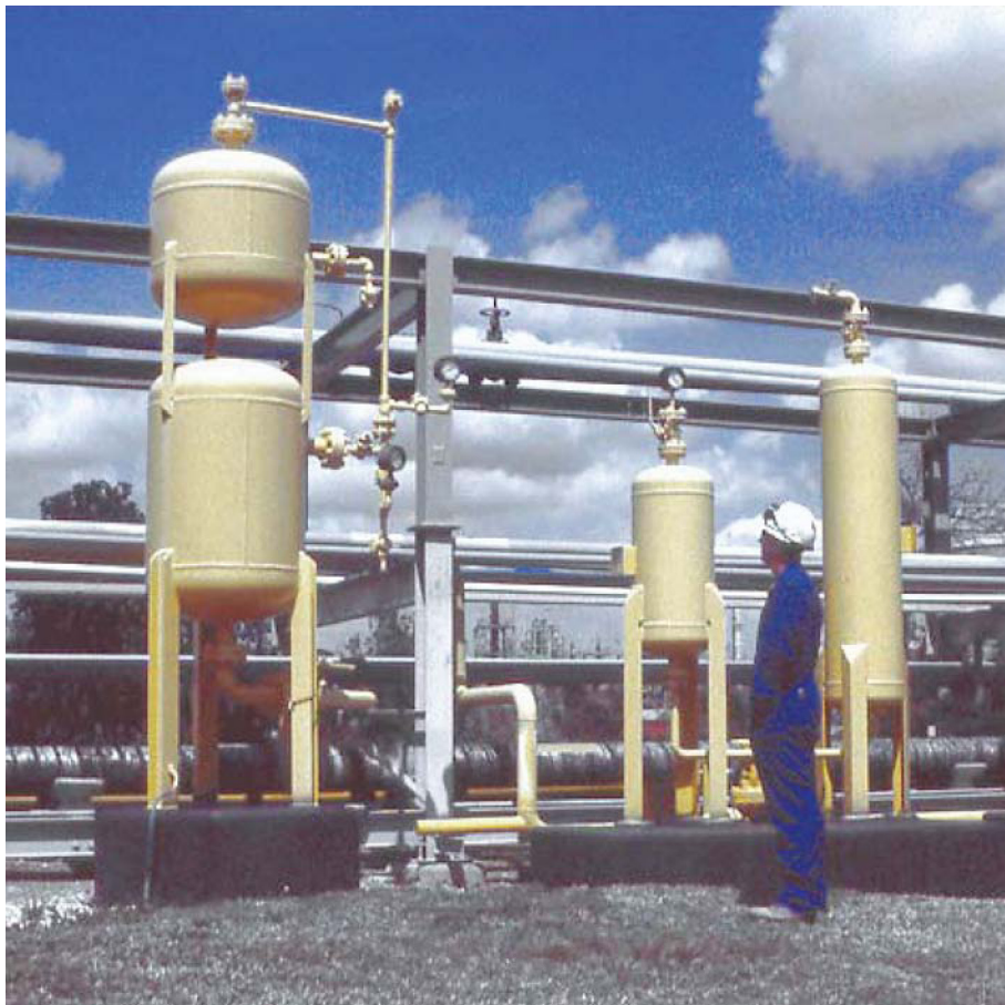
Figure 6.7 An engineer observes the pressure gauges on chlorine expansion bottles protecting liquid chlorine pipelines.
