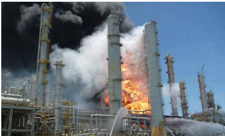
Figure 2.26 Hydrocarbon fire from a flawed review of a check valve substitution.
