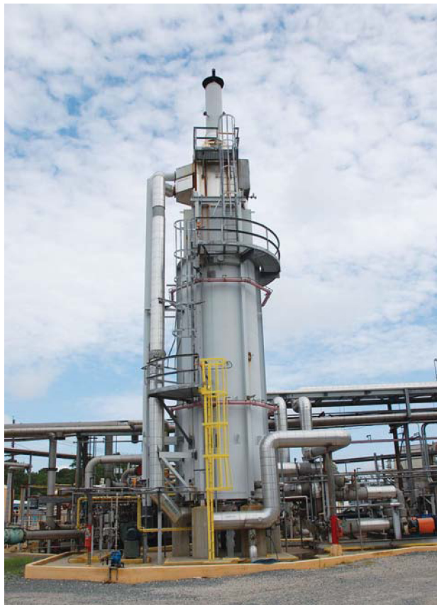
Figure 10.3 Today's hot oil heater with sophisticated safeguards to reduce failures.
