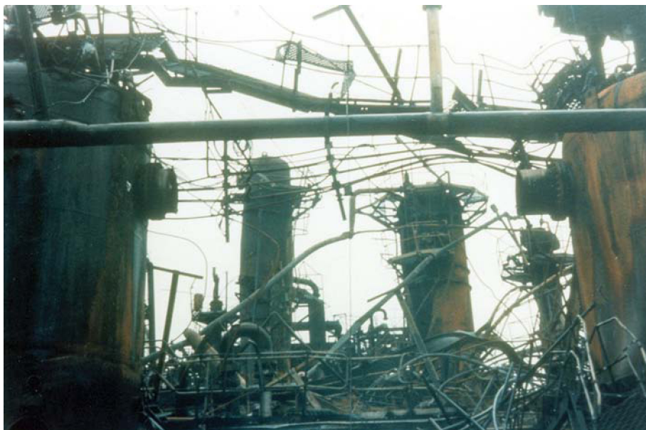
Figure 7.20 A destroyed section of the Flixborough reactor system. Photo Courtesy of Trevor A. Kletz.
