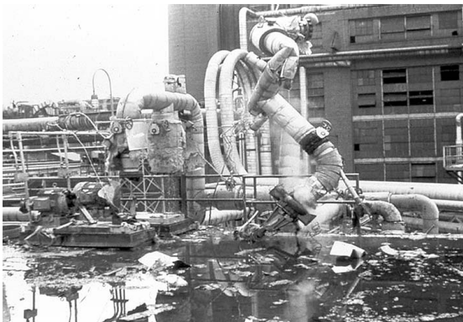
Figure 9.17 Condensate pump installation heavily damaged after operating with the suction and discharge valves tightly shut. Courtesy of Eastman Chemical Company.
