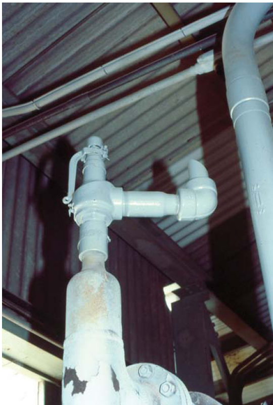
Figure 8.15 A threaded safety relief valve mistakenly reinstalled with a reduced discharge piping arrangement.
