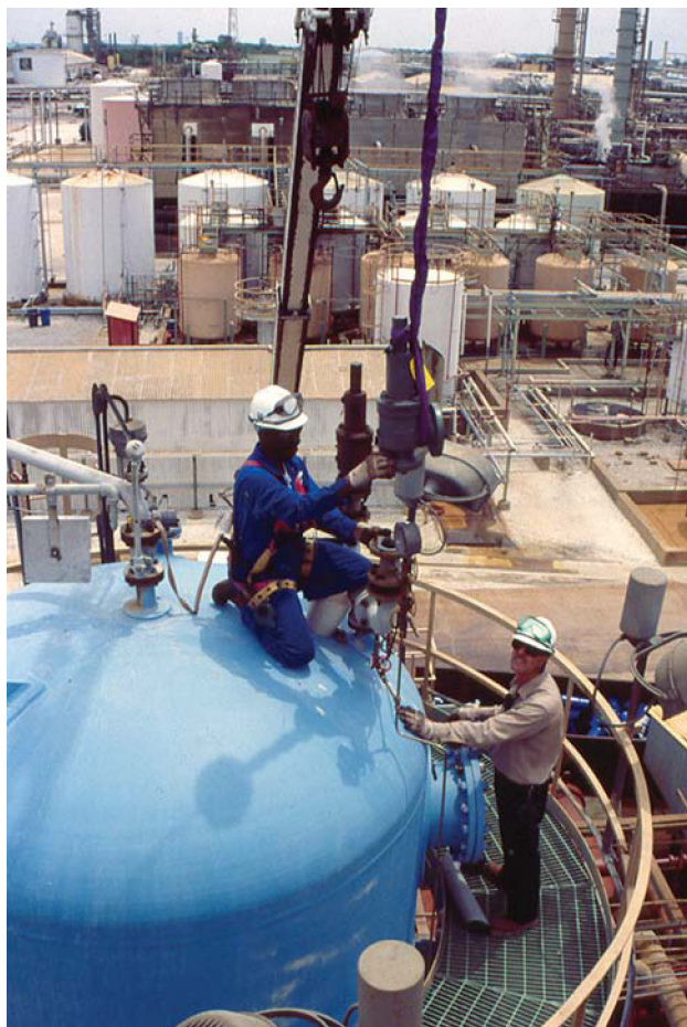
Figure 12.25 A crane is holding up a recently tested and reconditioned safety relief valve and mechanics are preparing to reinstall it in place on a reactor.
