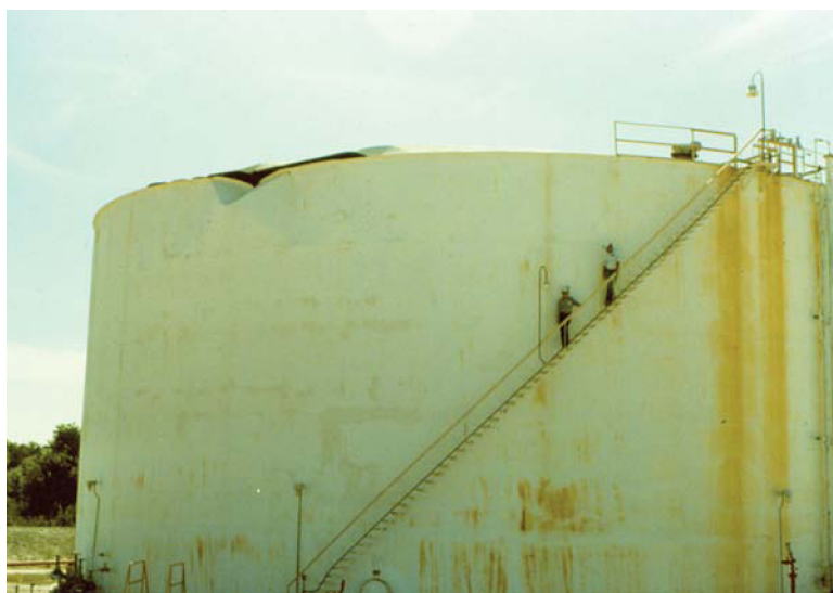
Figure 8.13 Overpressure problems created by a one-minute modification, a nitrogen pad protection system and changing weather.
