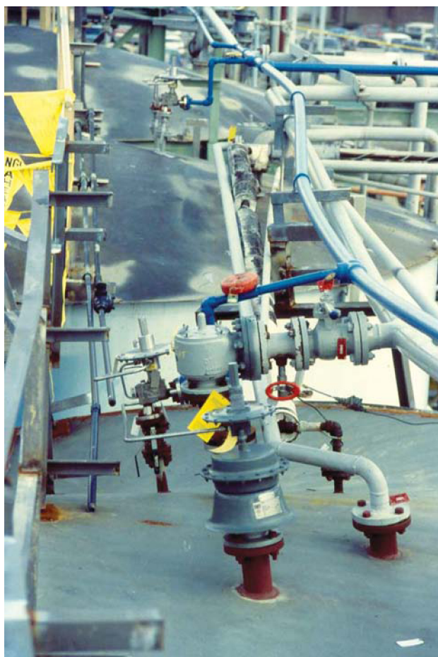
Figure 2.15 Newly installed but visually confusing piping system – after the incident.
