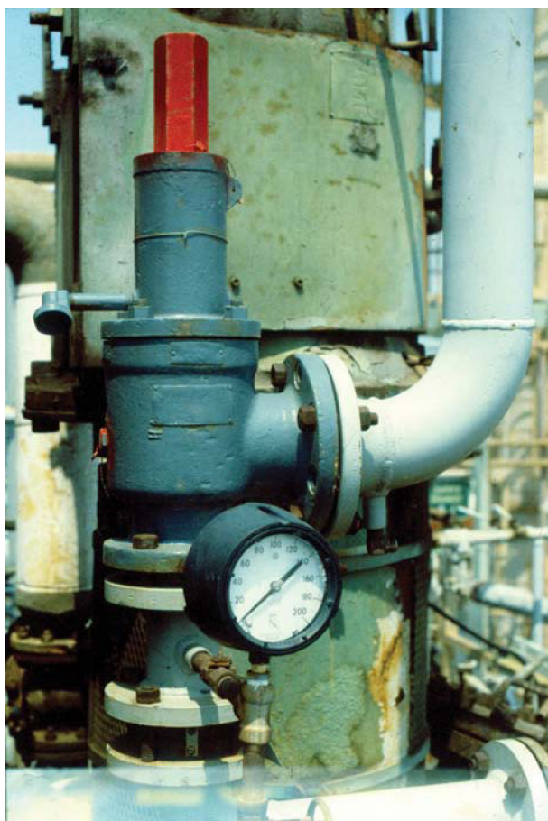
Figure 12.19 A typical safety relief valve, SRV, and rupture disc combination for a chemical process vessel. The rupture disk protects against the metal-to-metal seats on the SRV from seeping. The pressure gage lets you know if the rupture disk has “popped” or is leaking. The space between the rupture disk and SRV is required to be monitored by the ASME Code.
