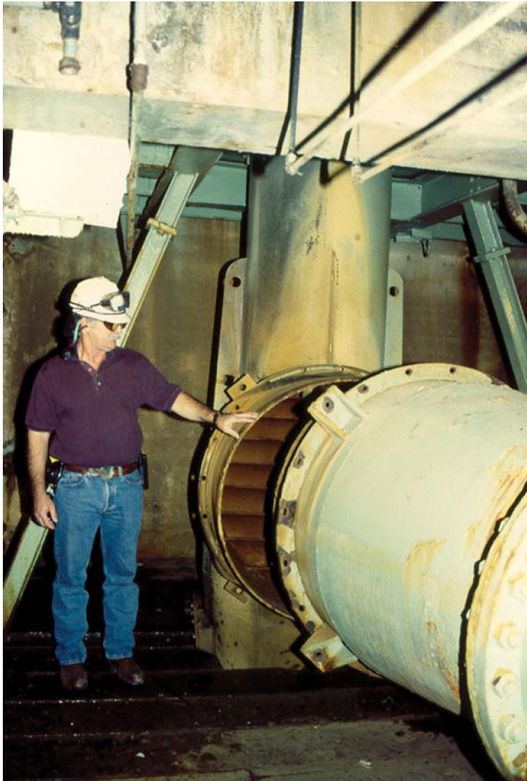
Figure 9.11 The force of the explosion thrust the base plate backwards and knocked the piping out of alignment.
