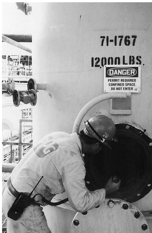
Figure 12.11 A vessel inspector makes an initial assessment of the vessel. He determines of any special inspection needs, such as ladders, scaffolding, mirrors, extra lighting, etc.
