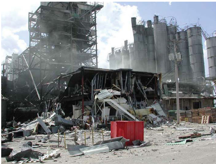
Figure 4.2 Destruction of Formosa Plastics two story safety and engineering offices. Courtesy of the U.S. Chemical Safety Board Report No. 2004-10-1-IL.
