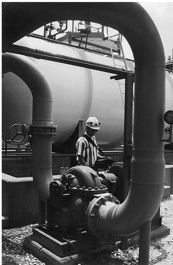
Figure 12.2 A vibration technician taking readings on a cooling water pump as part of a mechanical integrity program.
