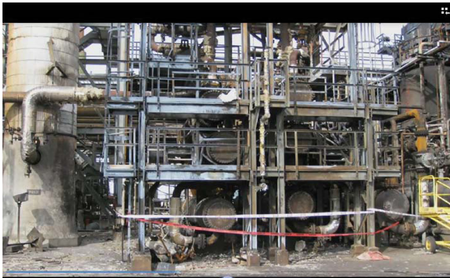
Figure 4.10 Tesoro's bank of burnt out heat exchangers.
