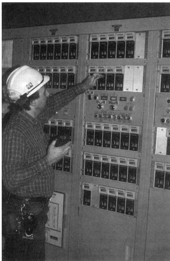
Figure 12.31 An instrument mechanic proof tests a critical instrument panel.
