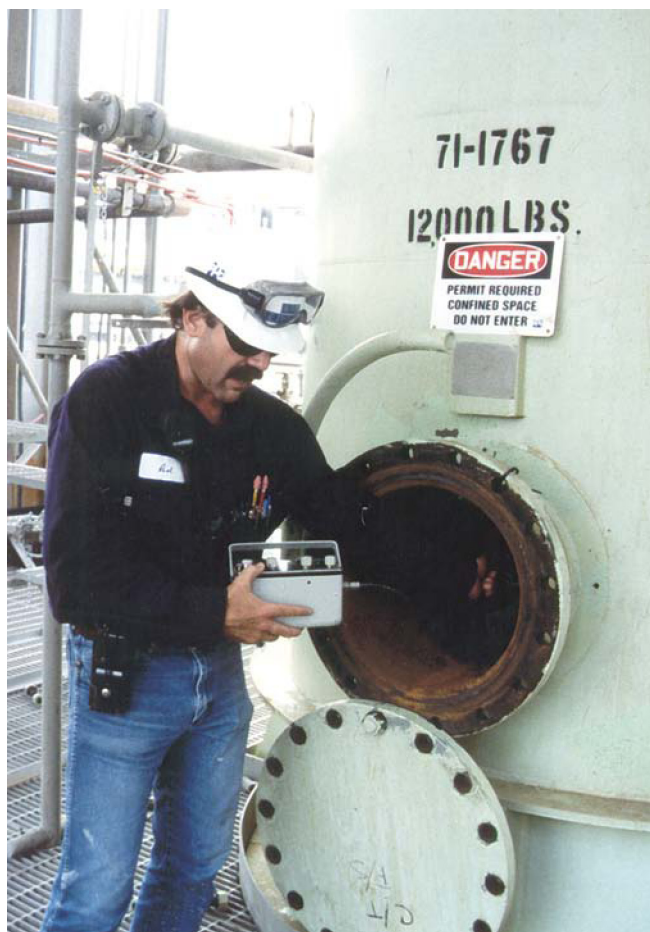
Figure 12.10 An operations foreman checks for proper blinding, proper drainage, washing and then checks the vessel's atmosphere prior to allowing vessel entry.
