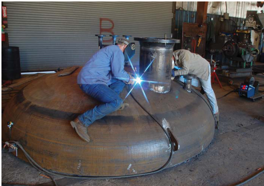
Figure 12.7 Metallic shop built vessels and components for vessel repair for hazardous materials must be constructed of certified materials employing code certified welders. New work and repairs must also be effectively tested.
