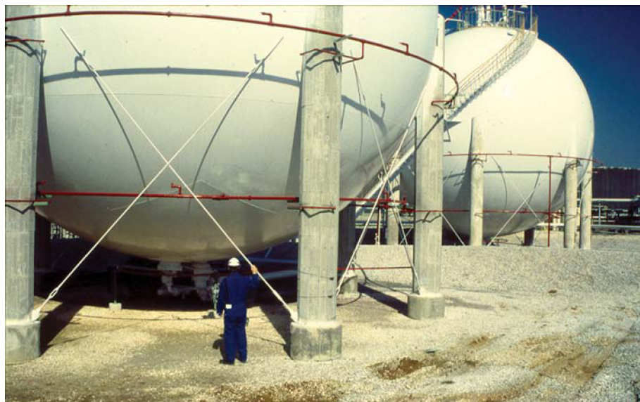
Figure 12.30 A chemical process operator witnesses the testing of an “emergency isolation valve” below a sphere, which stores a flashing flammable liquid.
