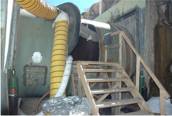
Fig. 20 Access door cut into confined space (penstock tunnel) at Xcel Energy hydroelectric plant (CSB, 2010b).
