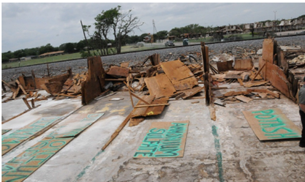
Fig. 19 Plywood bin walls in which FGAN (fertilizer-grade ammonium nitrate) and other fertilizer products were inappropriately stored at West Fertilizer Company (CSB, 2016b).
