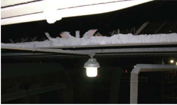
Fig. 17 Iron dust deposits on elevated surface at Hoeganaes Corporation facility (CSB, 2011).
