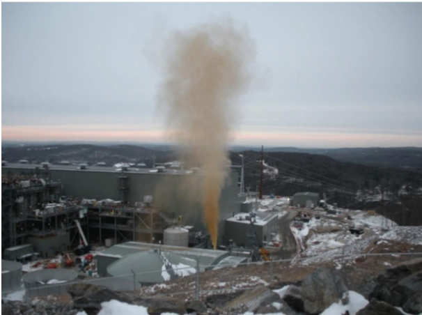
Fig. 16 Cleaning of fuel gas piping by gas blow at Kleen Energy site 1 week before incident (CSB, 2010c).
